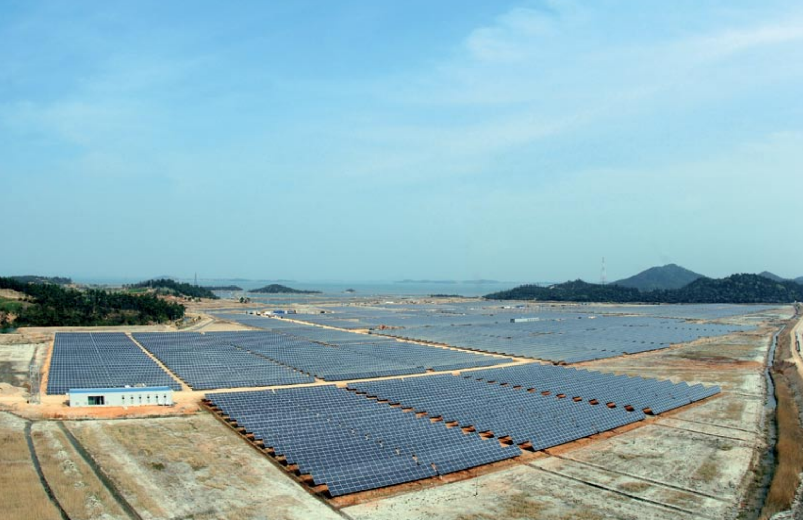
▲ Largest Asian PV power plant, Sinan, Southern Jeolla province, Korea, constructed in 2008 (courtesy: Conergy)
